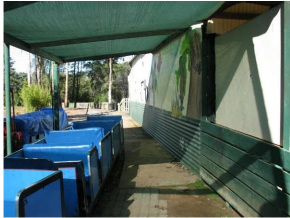
Figure: Eastern external wall of building.
