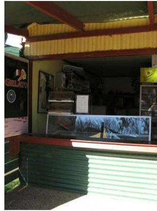
Figure: Shop front counter on northern side.
