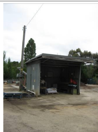
Figure: Smallest older shed.
