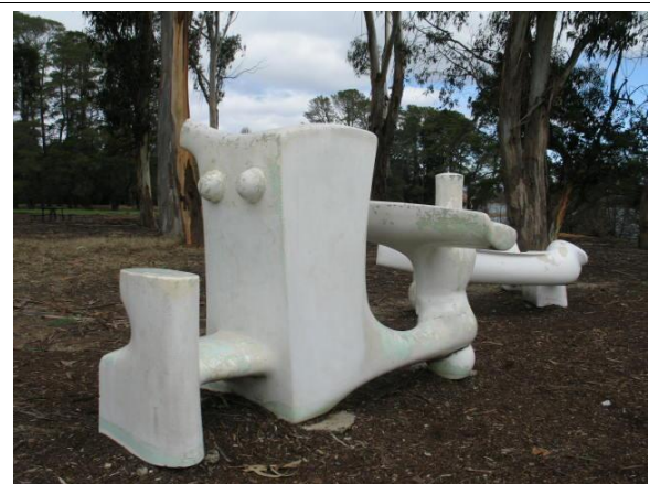
Figure: Closer view of sculpture with paint peeling.
