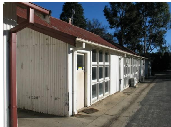
Figure: Southern end of Dispatch Office, laneway between buildings visible.
