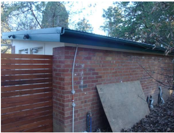
Figure: Toilet block on western side of Hobday's Cottage.
