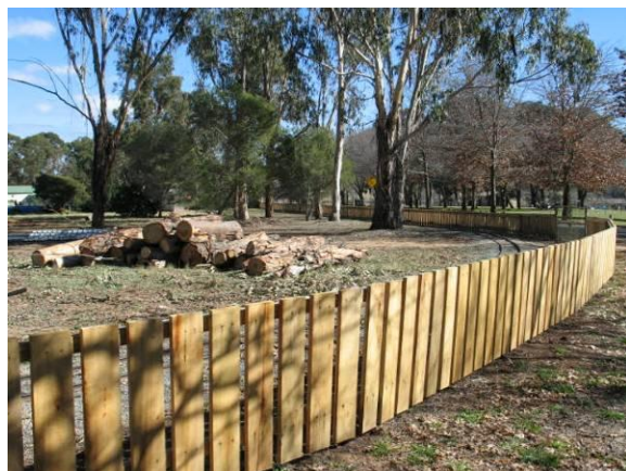
Figure: View of new fence between tunnel and station shop.
