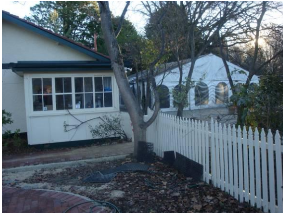
Figure: External view showing marquee on north side.
