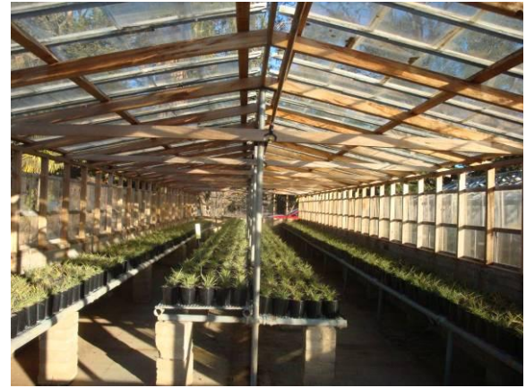
Figure: Interior of Glasshouse no. 25 showing brick pier shelving.
