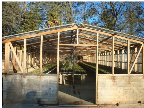
Figure: Glasshouse no. 25 with new timber frame.
