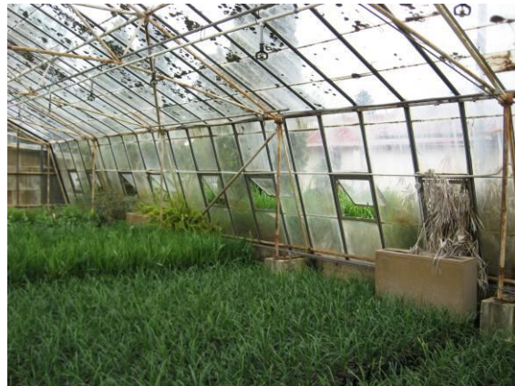
Figure: Interior of Display House.
