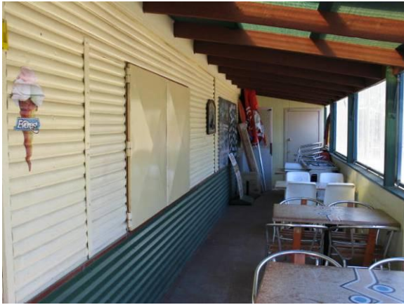
Figure: Interior of Verandah on western side of building.
