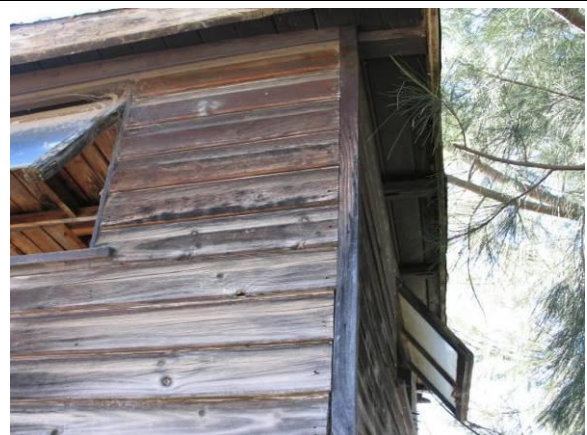
Figure: External view of timber cart, top-hinge windows visible.
