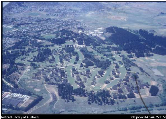
Figure B.7 Pre-lake Oblique Aerial, possibly 1950s or early 1960s (Source: National Library Australia nla.pic-an14324452-367-v Richard Clough Collection)
