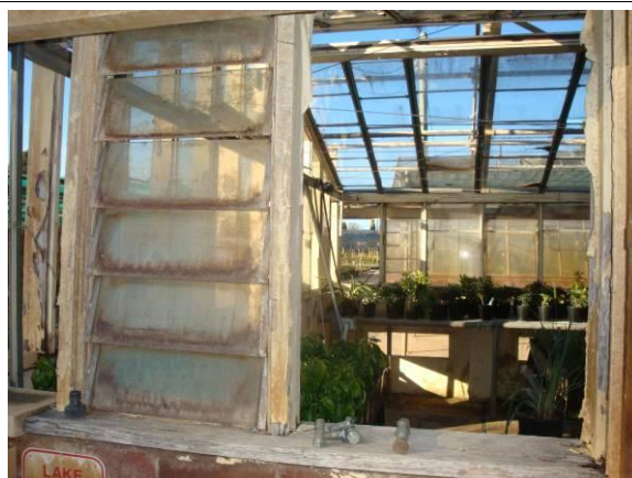
Figure: View into glasshouse no. 34 from western side.
