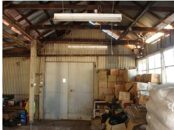
Figure: Interior of Dispatch Preparation looking north.
