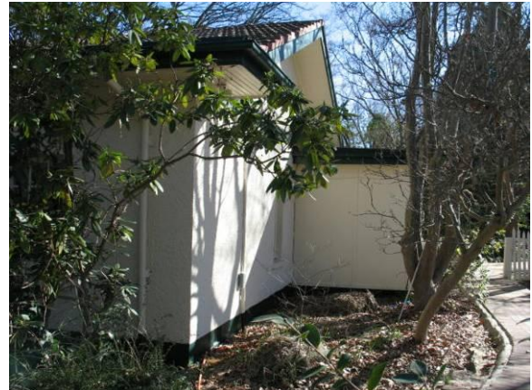
Figure: External view showing later addition on eastern side.
