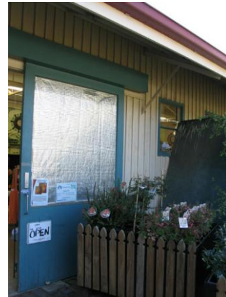
Figure: External view of western entry of main nursery building, showing timber clad exterior and top-rail sliding entry door.
