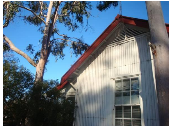
Figure: Northern end of Dispatch office.
