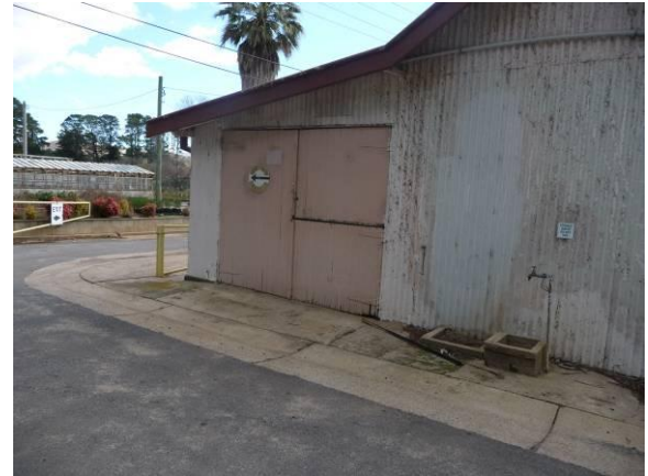
Figure: Southern end of Dispatch Preparation building showing Dutch entry door.
