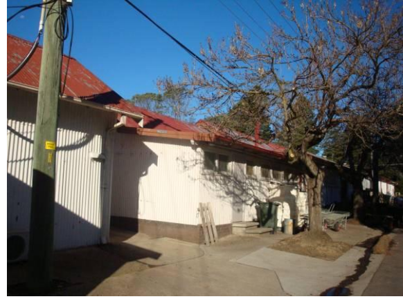
Figure: View of western, rear side of the building.
