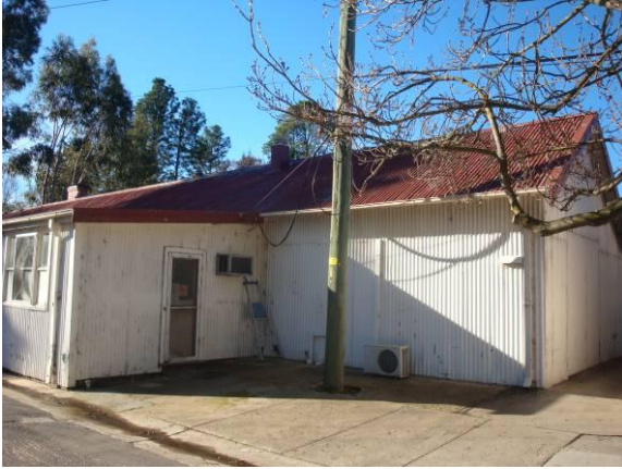
Figure: Rear, eastern side of Dispatch office showing lean to addition.
