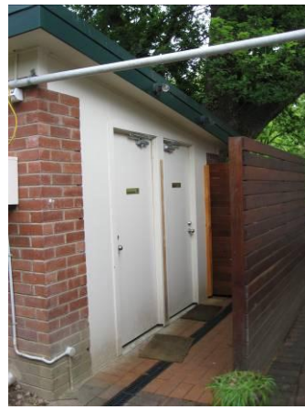
Figure: Toilet block entrance.
