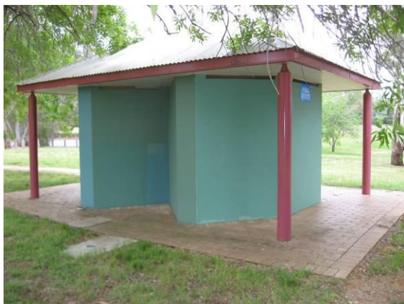
Figure: Rear of toilet block structure.
