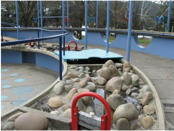
Figure: Detail of water feature with natural look rock bed and dam blocking system.
