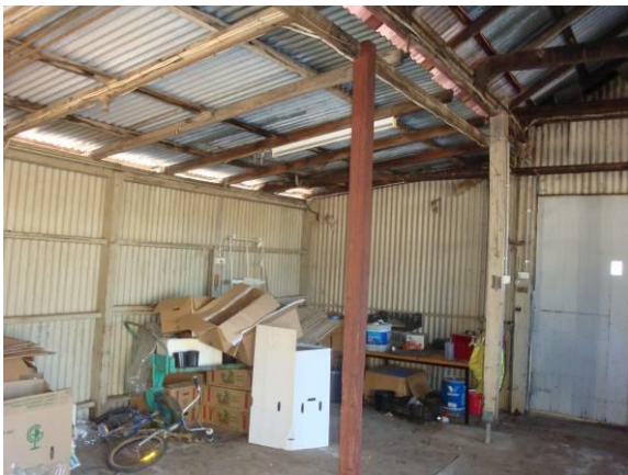
Figure: Interior of Dispatch Preparation showing new column supports.
