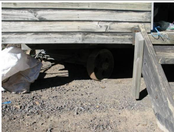
Figure: External view showing iron wheels support and timber stairs.
