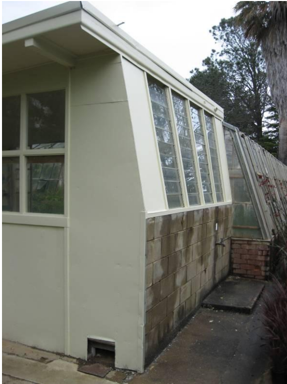
Figure: Western wall, showing glass louvres.
