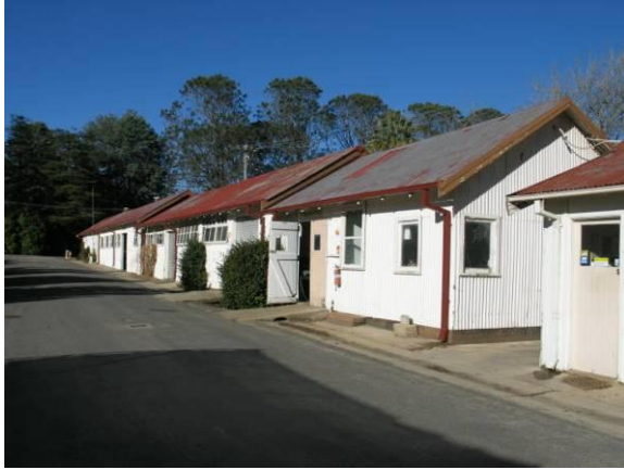
Figure: Row of three workshops, stepping up the site.
