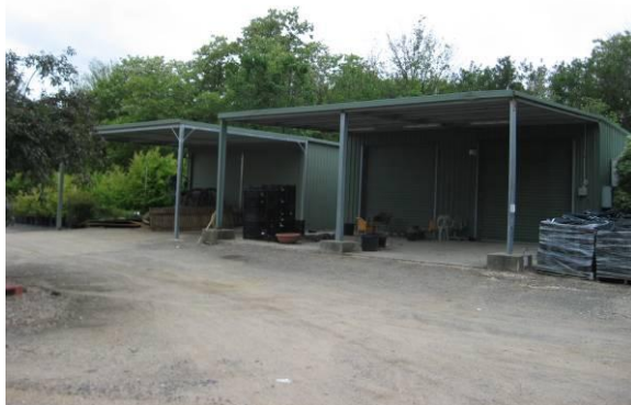
Figure: Two, double roller door sheds.
