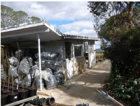
Figure: Building as it was in July 2010.
