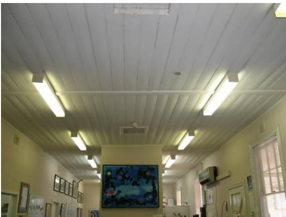
Figure: Interior ceiling of office space.
