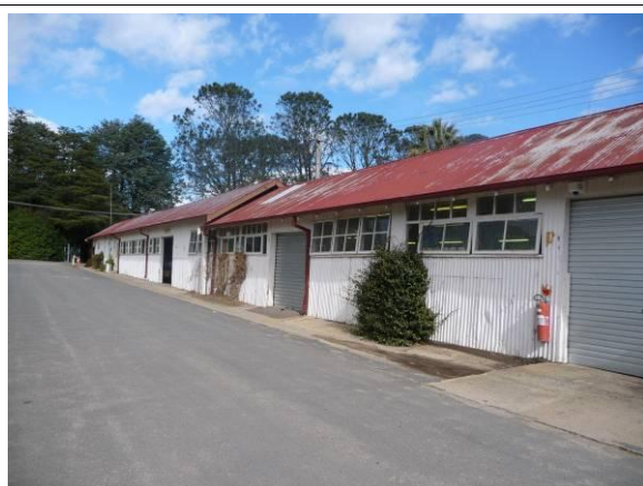
Figure: Main view of the Potting Shed, adjoining the Dispatch Preparation Workshop.
