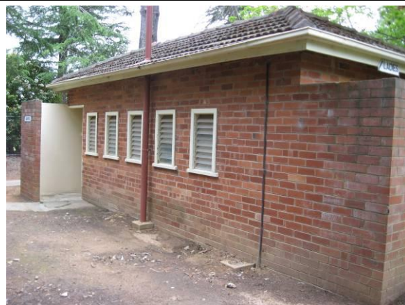
Figure: Western wall of toilet block.
