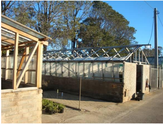
Figure: Glasshouse no. 26 with full height wall at front.
