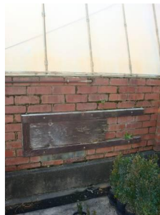
Figure: Timber ventilation panels on glasshouse no. 33.
