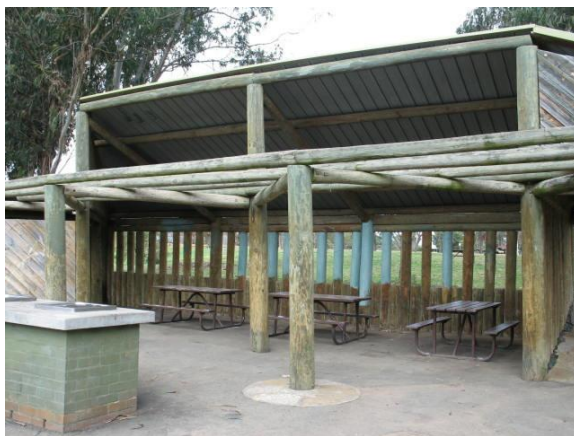
Figure: Front opening of shelter. Picnic tables and BBQ visible.
