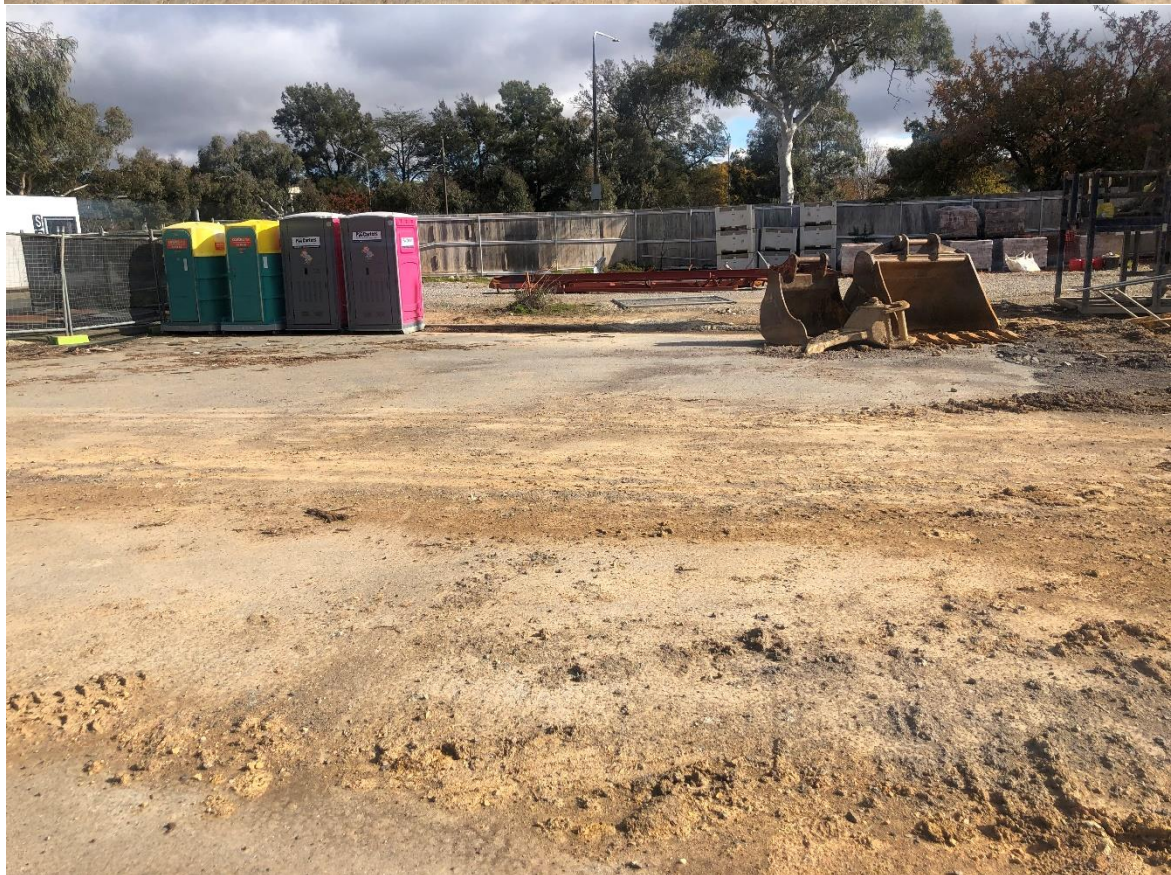
Photo 11 & 12. Existing condition of Karuah Street
