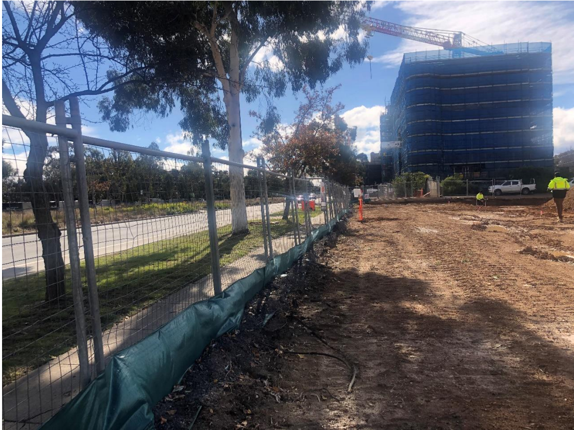
Photo.1 Existing Fench along the Northbourne Avenue
