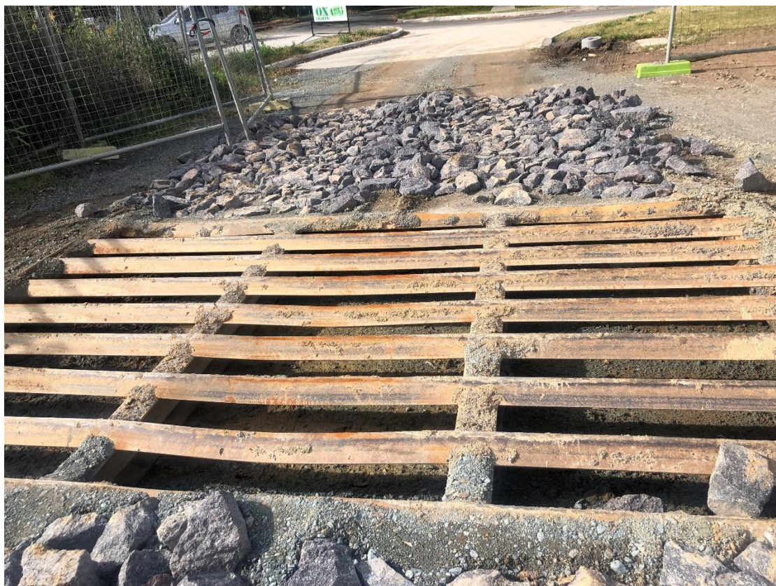
Photo 15. Existing Cattle Grate on the driveway to site (From Dooring Street)
