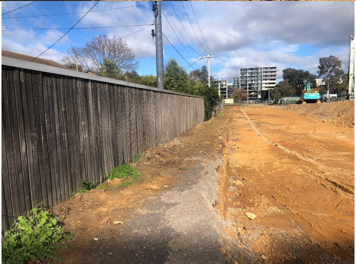
Photo 7 & 8. Existing fence along side houses of Lowrie Street
