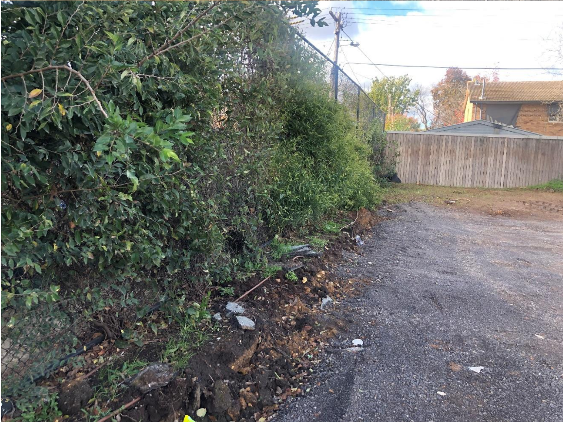
Photo 5 & 6. Existing fence along side the project p1.
