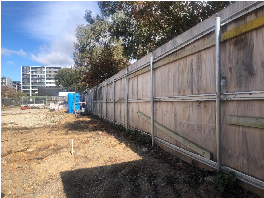
Photo.2 Existing Fench along the Northbourne Avenue
