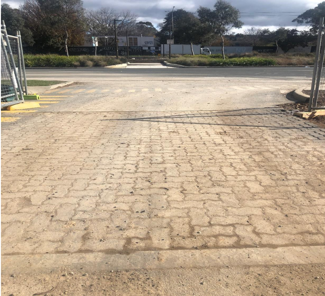
Photo 3 & 4. Existing driveway from Northbourne Avenue
