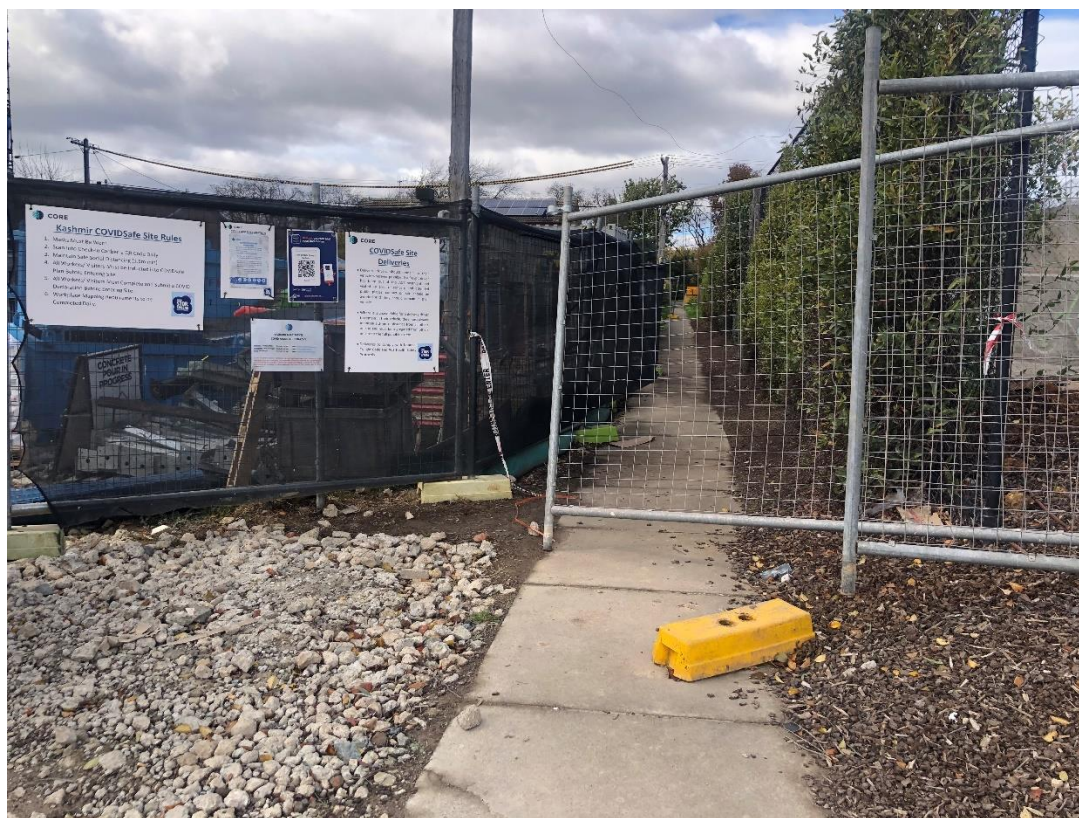
Photo 18. Existing footpath near driveway from Northbourne Avenue
