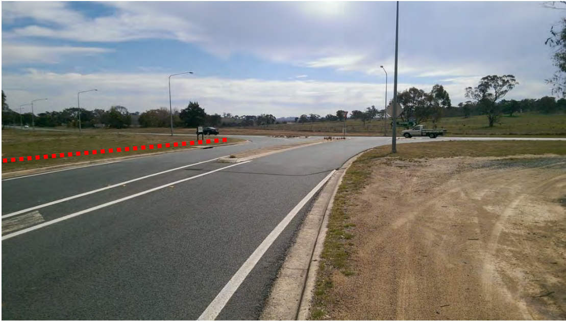
Photo 4.7: Owen Dixon Drive at T-Intersection with Kuringa Drive, looking North, with proposed shared path construction shown in red.
