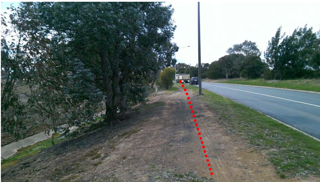
Photo 4.2: Kuringa Drive looking North/East, showing the open concrete drain on the left. The future alignment of the shared path shown in red dashed line.
