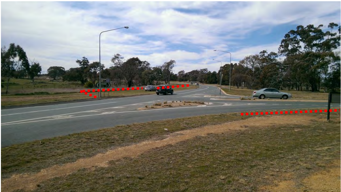
Photo 4.8: Kuringa Drive looking East to T Intersection with Owen Dixon Drive intersection on right hand side, proposed shared path detailed in red.
