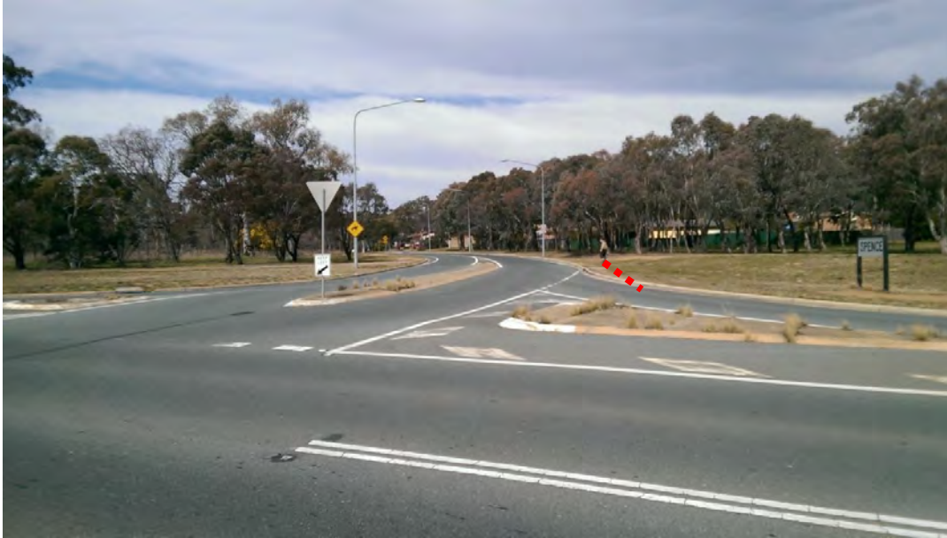
Photo 4.9: Kuringa Drive and Owen Dixon Drive T- Intersection, looking South. The existing street lights and concrete medians/refuge islands are shown on the intersection.
