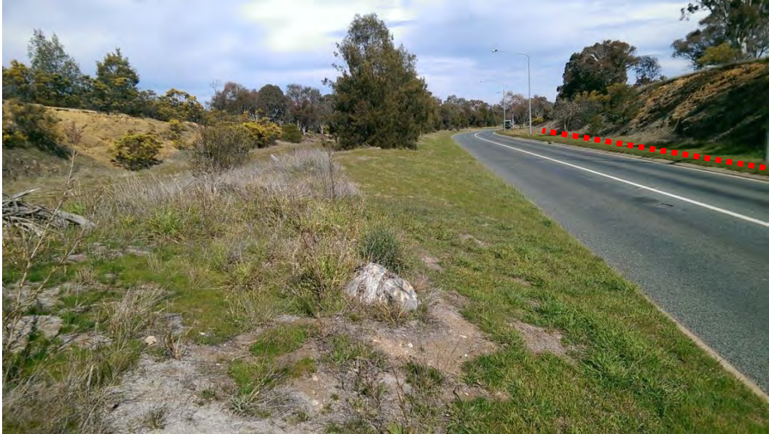
Photo 4.5: Kuringa Drive looking South/West. The earthworks formation is shown on the left to allow future duplication of Kuringa Drive on left hand side and future shared path alignment is shown by red dashed line.
