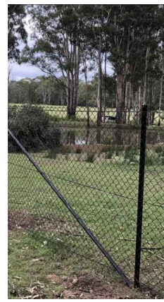
FE1 1.8M HIGH CHAIN LINK FENCE
