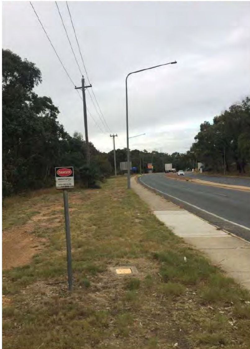
Figure 4-17: Energy utilities on the eastern side of Haydon Drive
