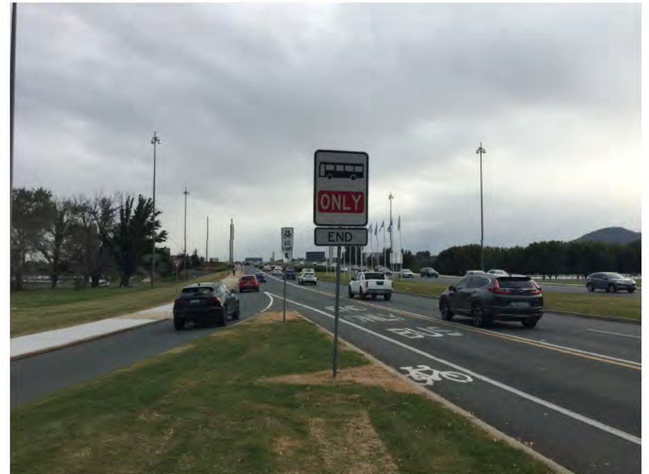
Figure 4-8: On Commonwealth Avenue northbound the bus lanes finish just before the Commonwealth Avenue Bridge
