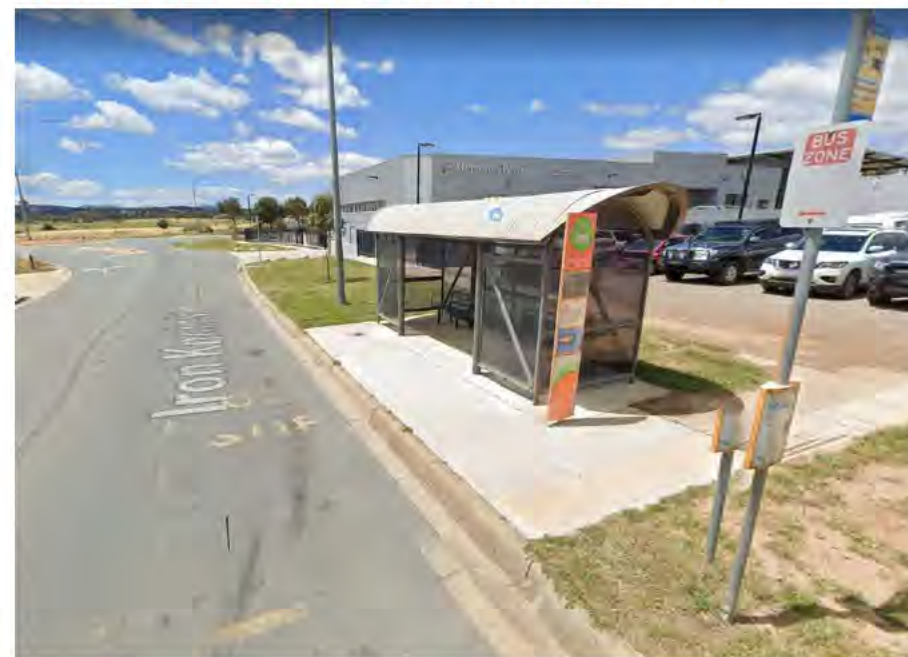
Figure 6-21: Fyshwick Park and Ride stop in Iron Knob Street
