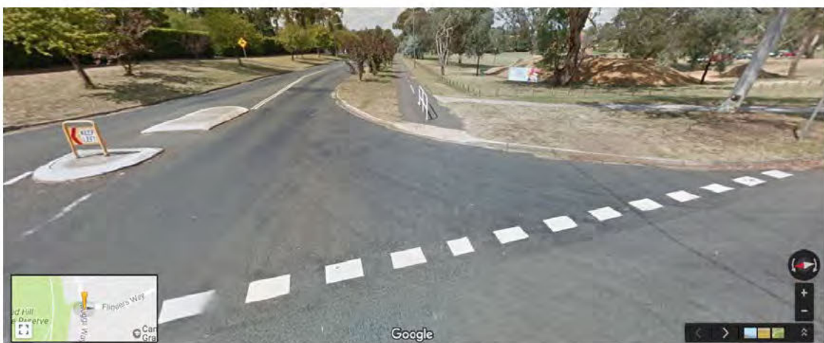
Figure 5 – Streetview – existing kerb ramp directs users into the intersection and into the area of turning cars
