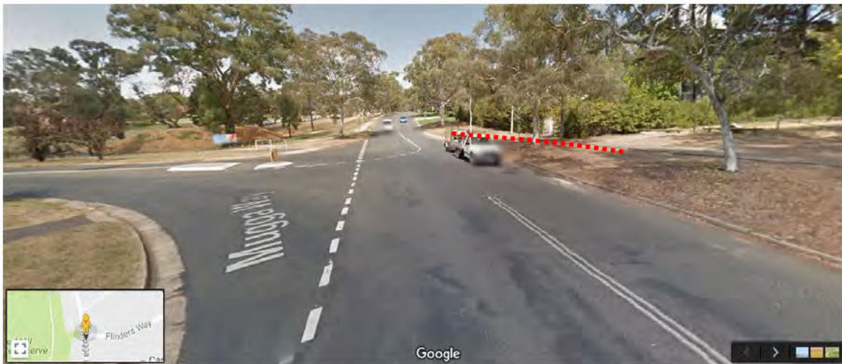
Figure 2 – Streetview – Proposed path near intersection of Flinders Way
