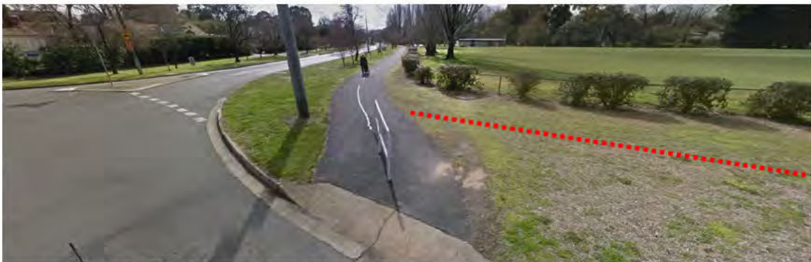
Figure 5 – Streetview – Existing off-road shared path on Flinders Way
