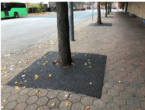
Tuggeranong Bus Interchange - New Root Pave product has been contoured over existing structural tree roots and trip hazards have been eliminated.
