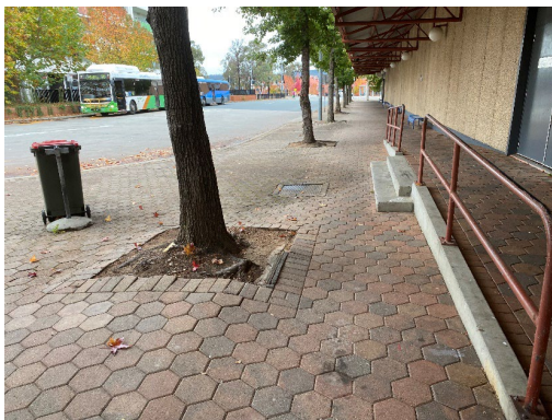
Tuggeranong Bus Interchange - New Root Pave product has been contoured over existing structural tree roots and trip hazards have been eliminated.
