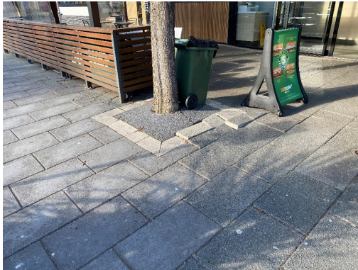
Amaroo Shops – Root Pave product finished level with surrounding concrete pavement. Root Pave product has a high porosity rate, is flexible and trafficable.
