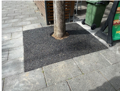
Amaroo Shops – Root Pave product finished level with surrounding concrete pavement. Root Pave product has a high porosity rate, is flexible and trafficable.
