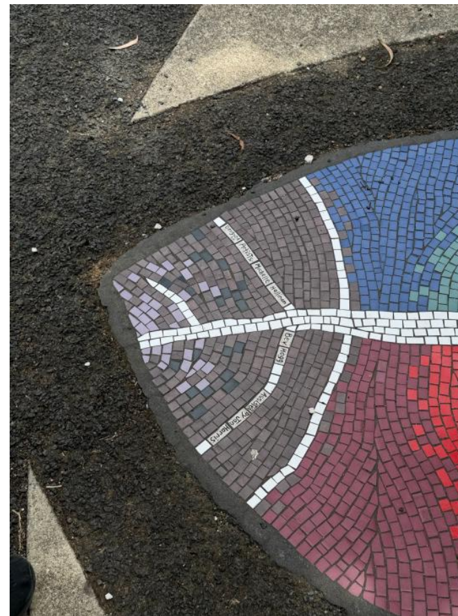
Retain and refurbish existing mosaic paving
