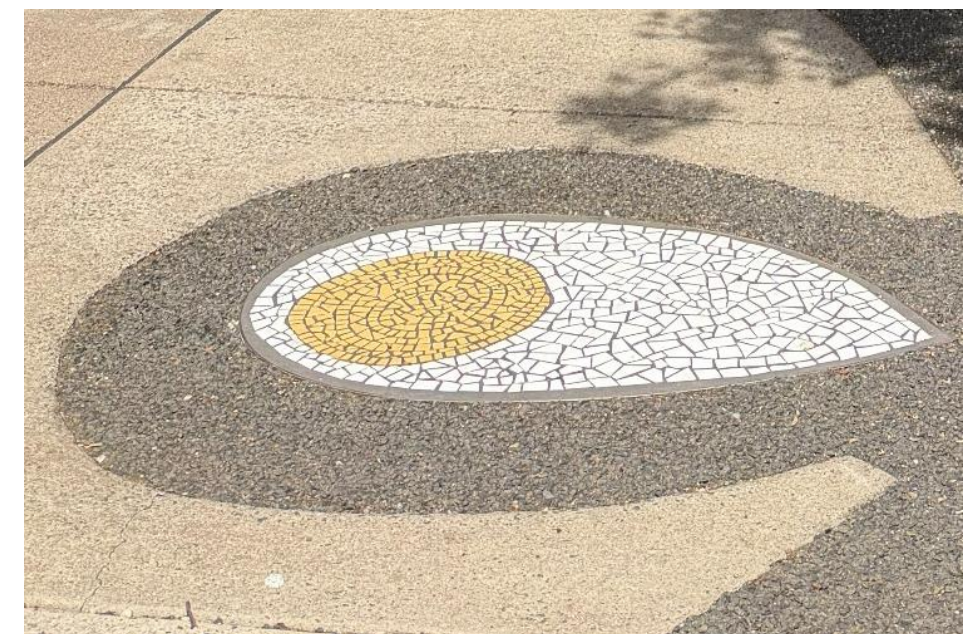
Retain and refurbish existing mosaic paving
